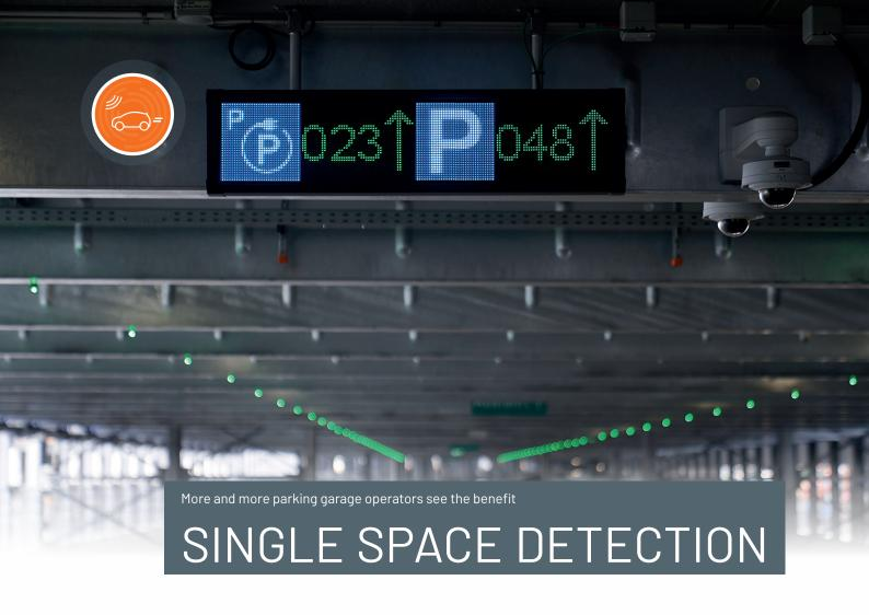
Our pilot project in Frankfurt/Main has become a place of pilgrimage for parking garage owners and operators. There, for the first time, we installed LOBO, the dynamic parking guidance system, with its single-space detection feature. This system offers brand new possibilities for efficient management of available parking spaces.
